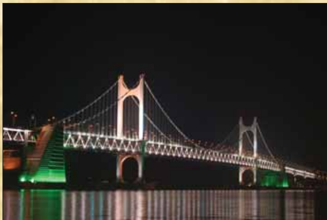
Figure 1 - Gwangsan Bridge at night, Busan, South Korea.
